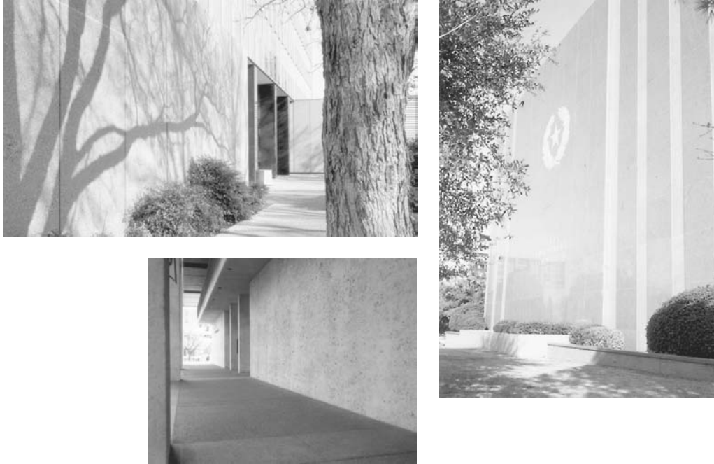
Figure 5-12 Stone veneer slabs.
