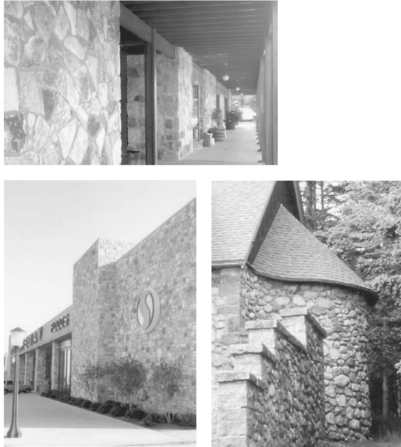
Figure 5-11 Rubble stone veneers.
